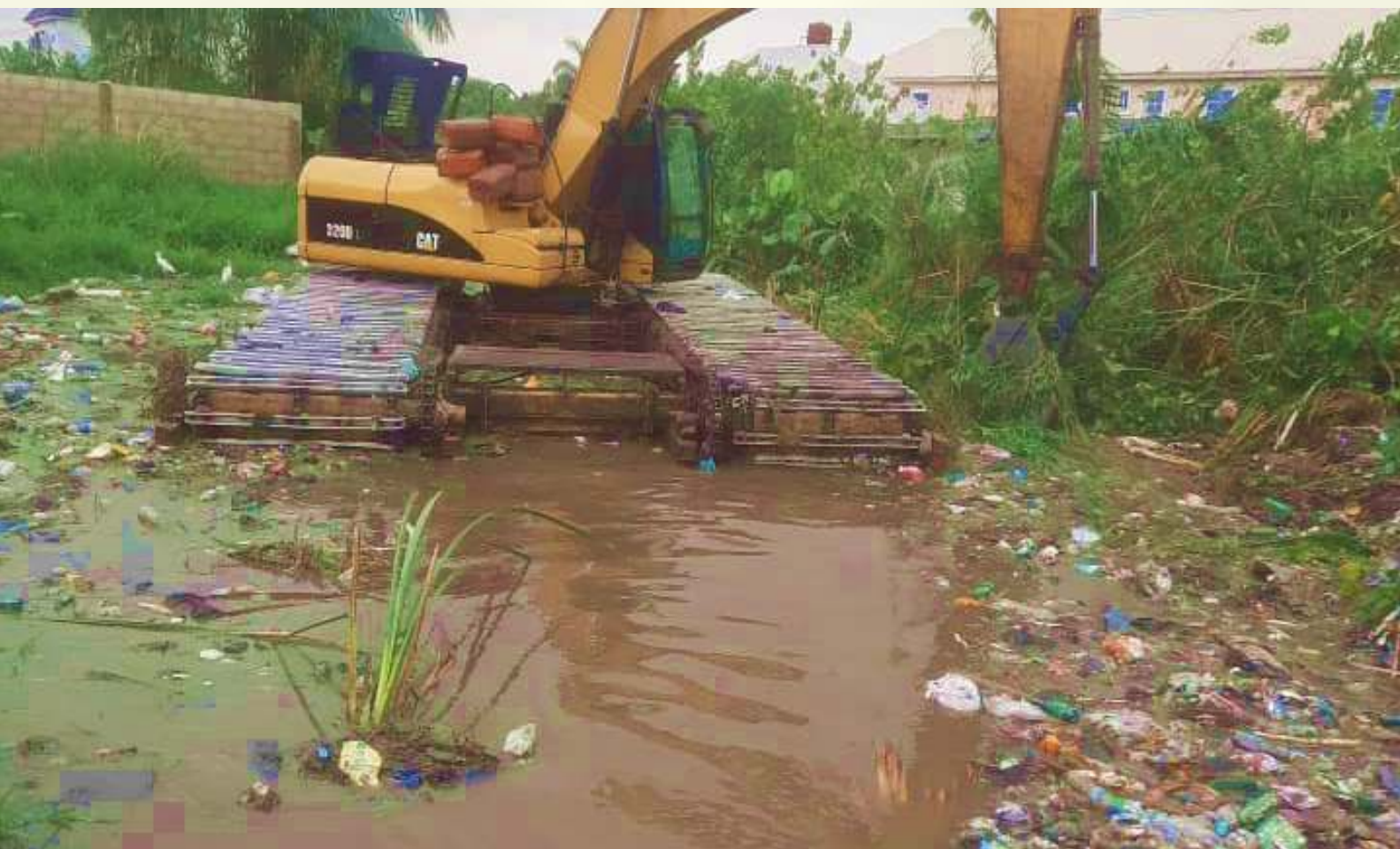
📍 IGBOJIA CANAL DURING THE CHANNELIZATION EXERCISE
