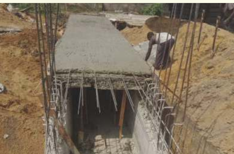
CONSTRUCTION OF BOX CULVERT AT OGUNFAYO
